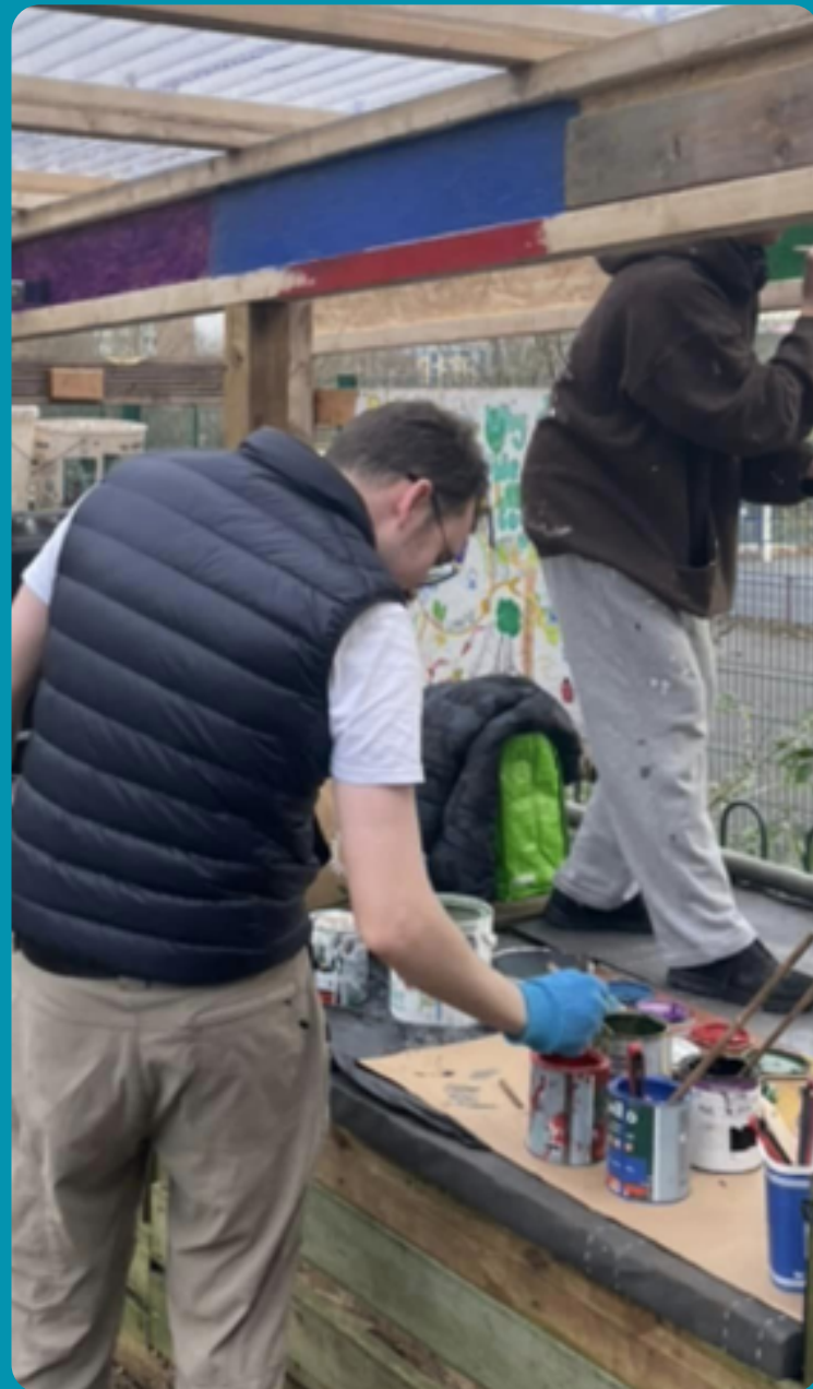
Dame Emily - Renovating the compost bin
